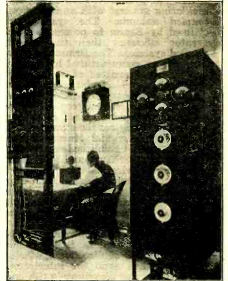
Fig. 3. Main control panels of a Radio Broadcast Station.
